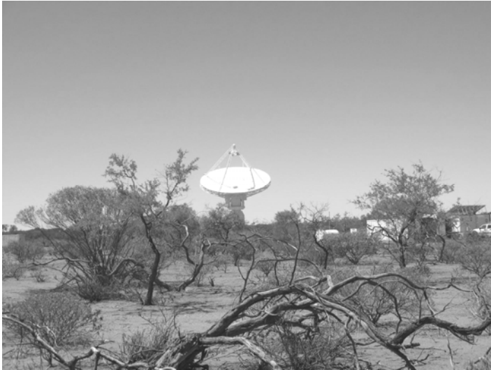
The first ASKAP antenna erected in the West Australian outback undergoes testing, prior to the arrival of 35 similar antennas to which it will be electronically linked. Image credit: Dave DeBoer, CSIRO.
