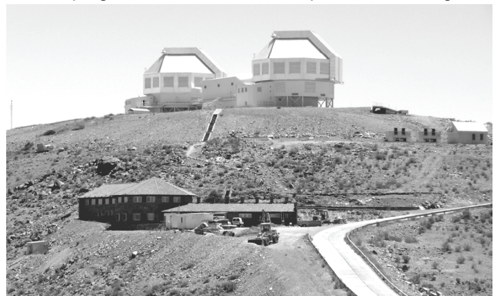
The twin "domes" of the Magellan telescopes feature large louvres which are opened at night to help keep the air around the telescopes at the same temperature as the outside air and preserve the excellent seeing.
