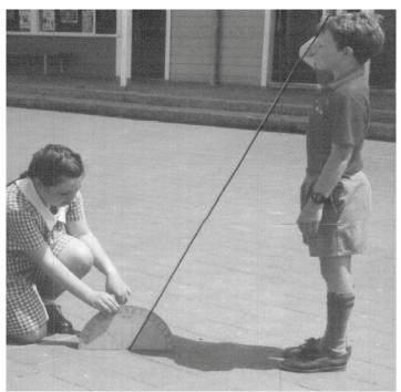
Measuring the altitude of the Sun: does it suggest a way of measuring the height of a tree or even a building? This experiment offers many possibilities!
