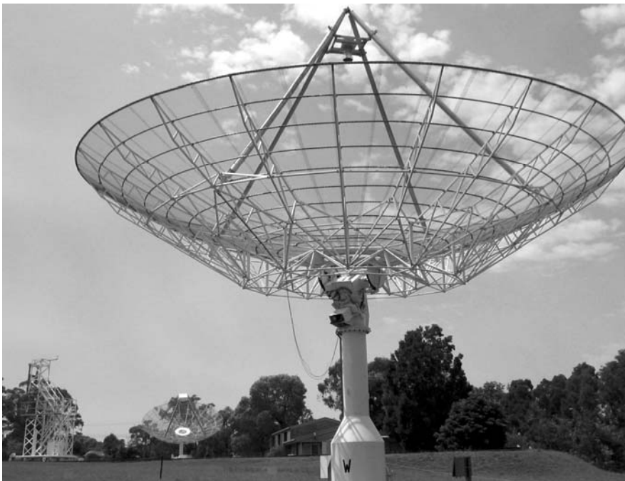
Two of the 13.7m diameter dishes recovered from the Fleurs Synthesis Telescope, back in operation as the Australian New Technology Demonstrator for the Square Kilometre Array. The antenna in the background has a focal plane array (the large square package suspended above the dish), while the foreground antenna has just a single receiver.
