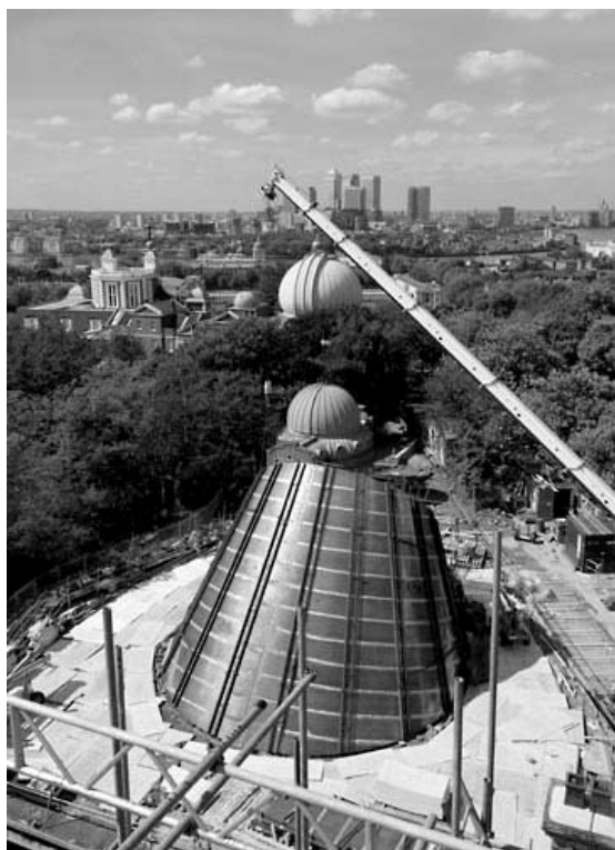
The photo shows the exterior of the Peter Harrison planetarium with bronze cladding in place
