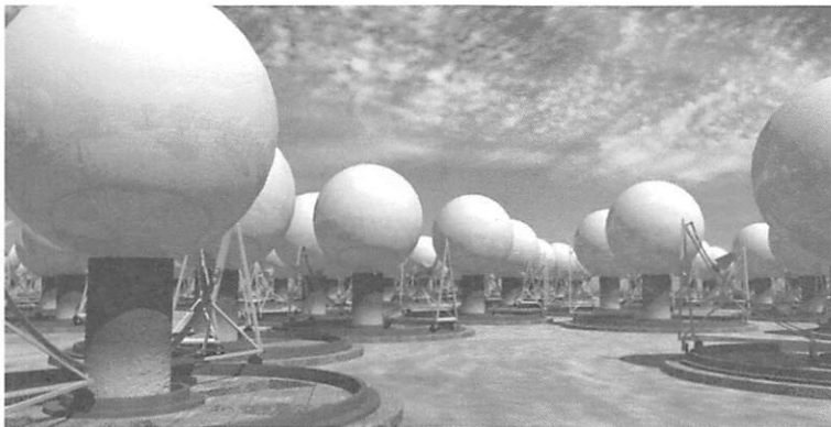
Computer visualisation of what an array of Luneberg Lenses in Western Australia might look like, if selected as the antenna design for the SKA. (Image: courtesy of Chris Fluke, Swinburne University of Technology.)
